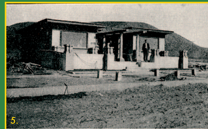
TYPICAL STRAND HOME UNDER CONSTRUCTION
