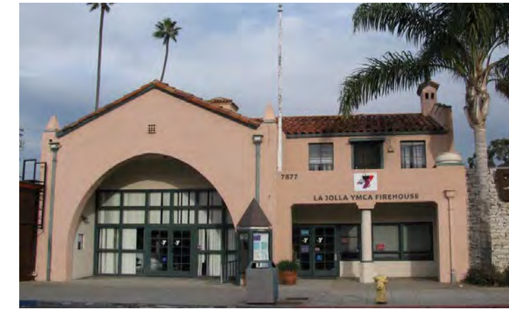
7877 Herschel Ave. La Jolla Fire Station Engine Company 13 HRB# 164 1937 Mission Revival Spanish Eclectic
