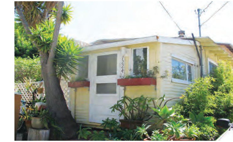
7224 1/2 Fay Ave. John Meed Ray Cottage HRB# 1155 1918 Cottage
