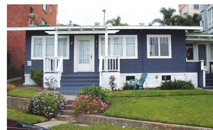
1046, 1049 & 1051 Coast Blvd. F.M. Sheppard Duplex and House Rentals HRB# 708 1911 Craftsman
