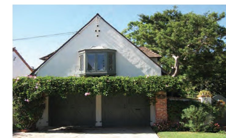
7148 & 7150 Monte Vista Ave. Morgan-Larkins-Marrone Residence HRB# 226 1935 Tudor, Edgar Ullrich
