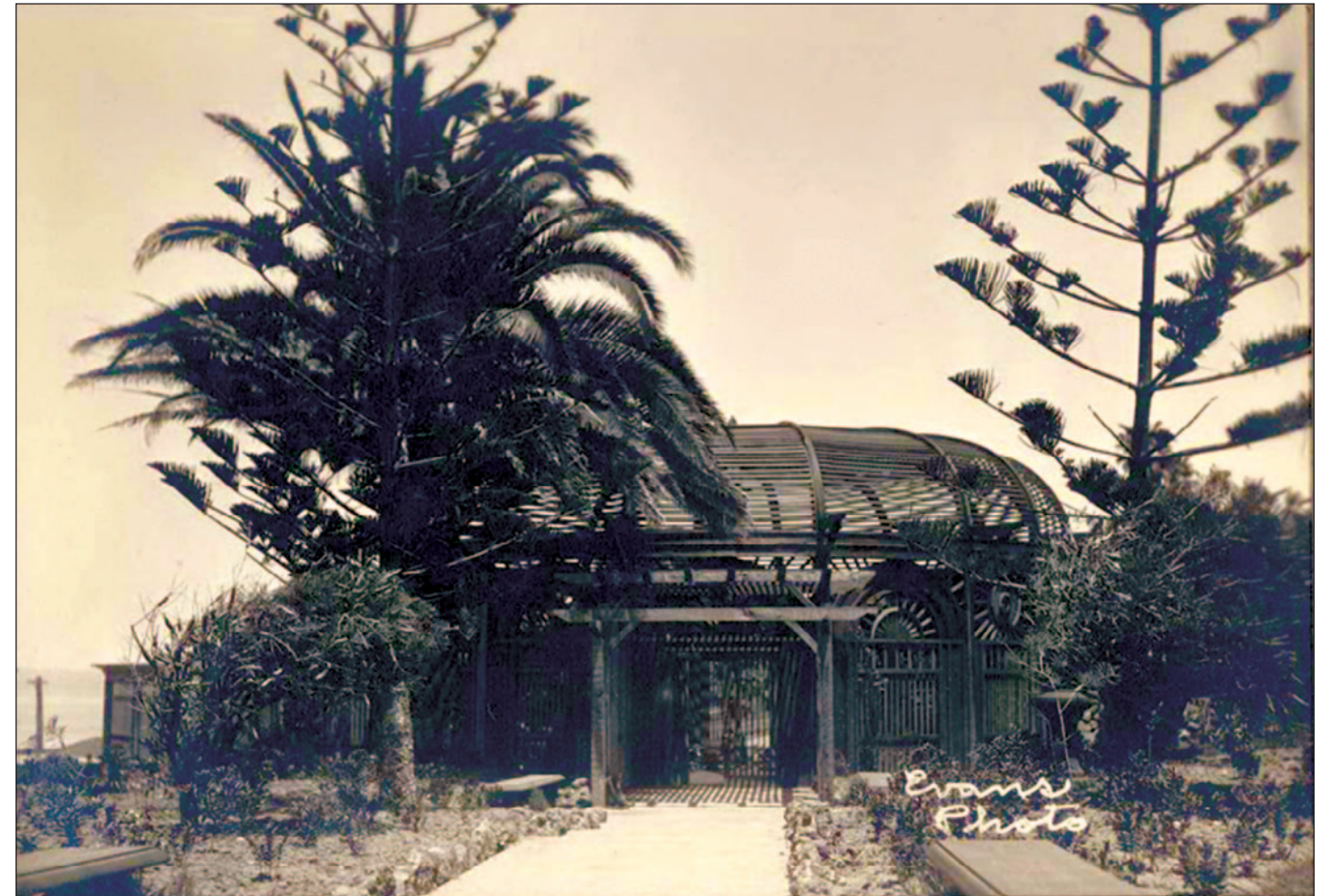
Built in the shape of a rotunda, Ellen Browning Scripps' lath house, above, was flanked by large pine trees. Interior, left, show symmetrical design of plantings with a small lily pond at the center.
