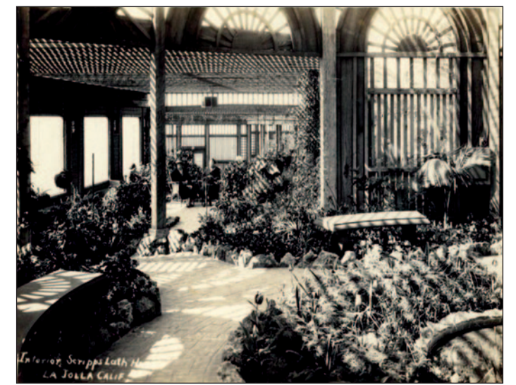
With a light-bathed interior and semi-transparent use of materials, the pergola was built site-specific to its views of the ocean
